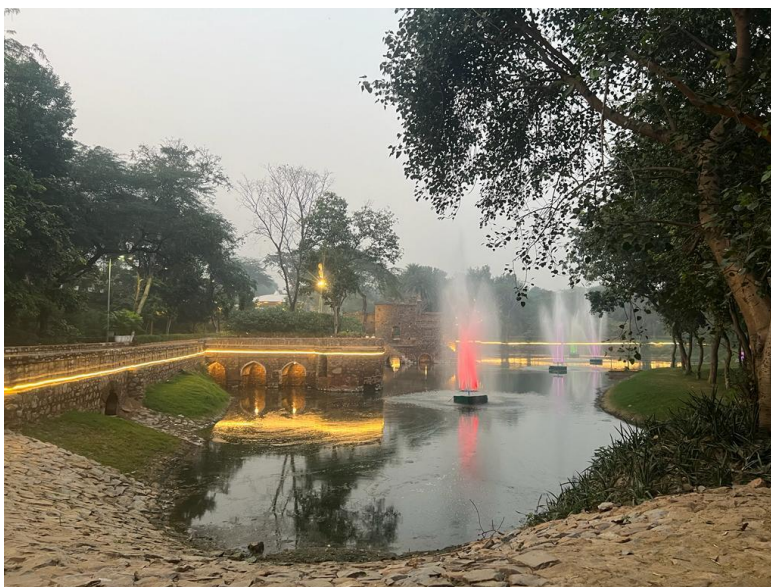
Figure 7: Side View of Water-body and lighting
