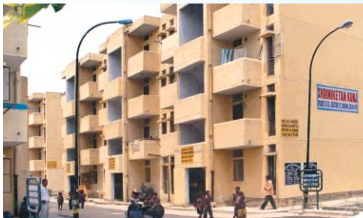
LIG Flats at Rohini
