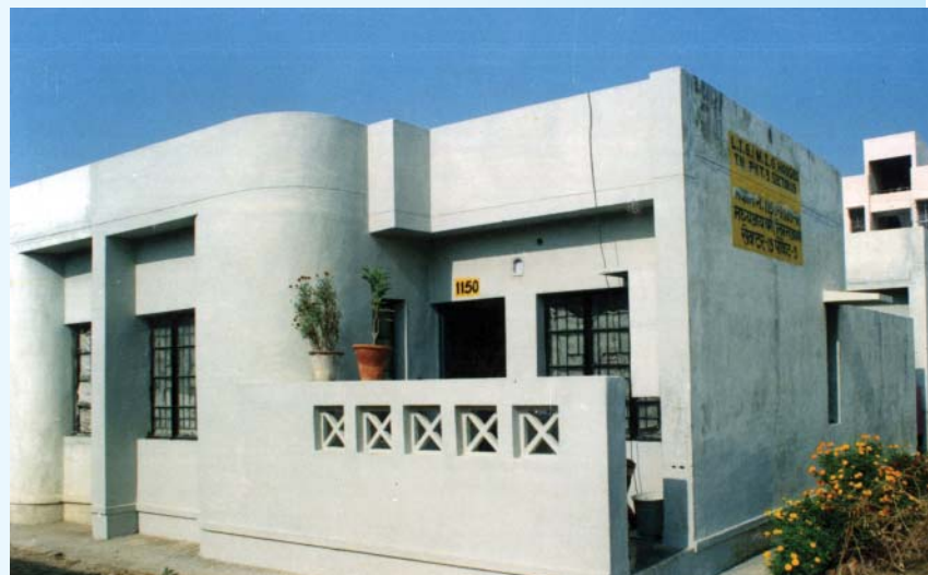
EWS Houses at Bindapur
