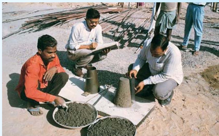
Quality Control Test being conducted on-site
