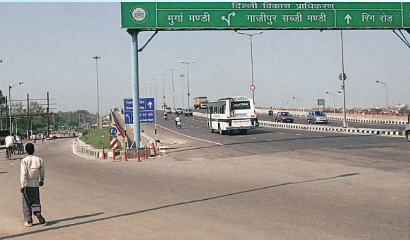
Flyover constructed by DDA at Ghazipur Subzi Mandi
